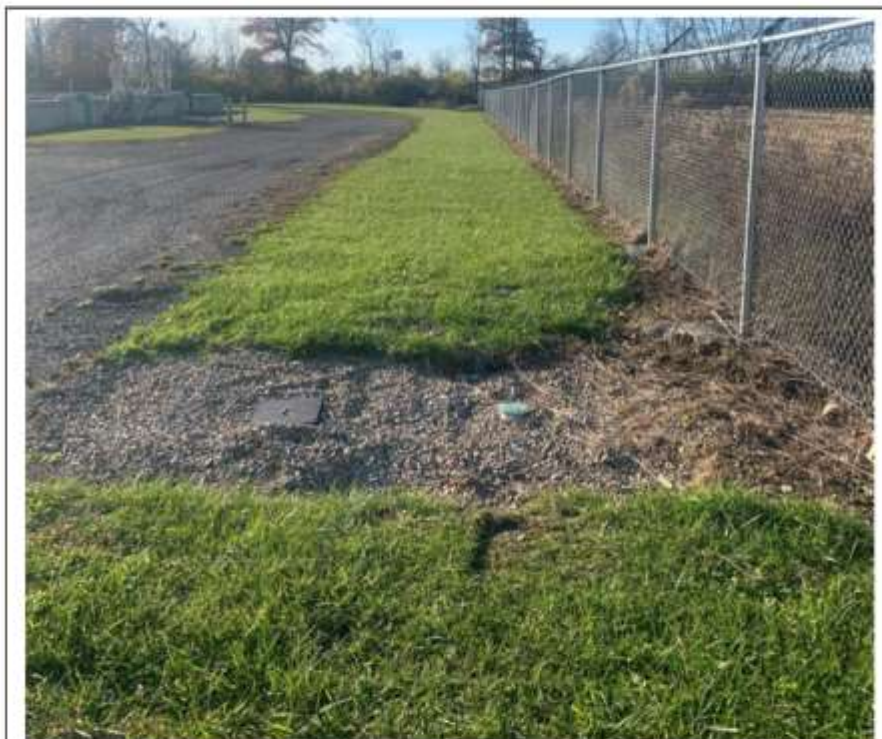
Figure 3.01-1 Existing North Stormwater Ditch
