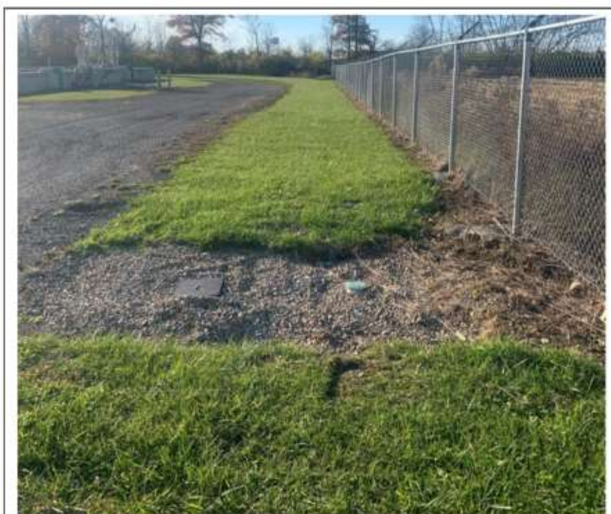
Figure 3.01-1 Existing North Stormwater Ditch
