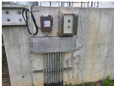
RAS & WAS Splitter Structure
