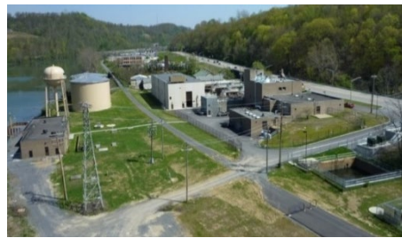
MUB's Water Treatment Facility (2013).
