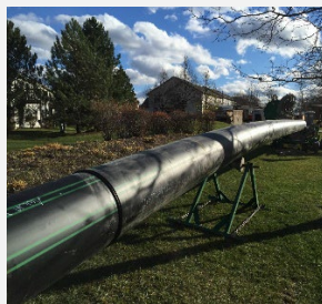
Unique design challenges can be met using trenchless pipe installation.
