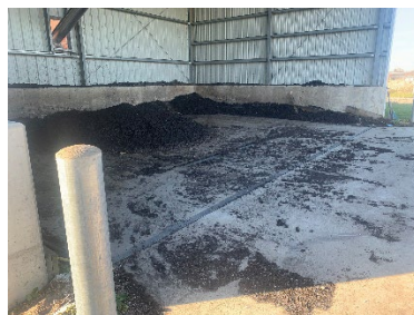
Sludge Cake Pad
