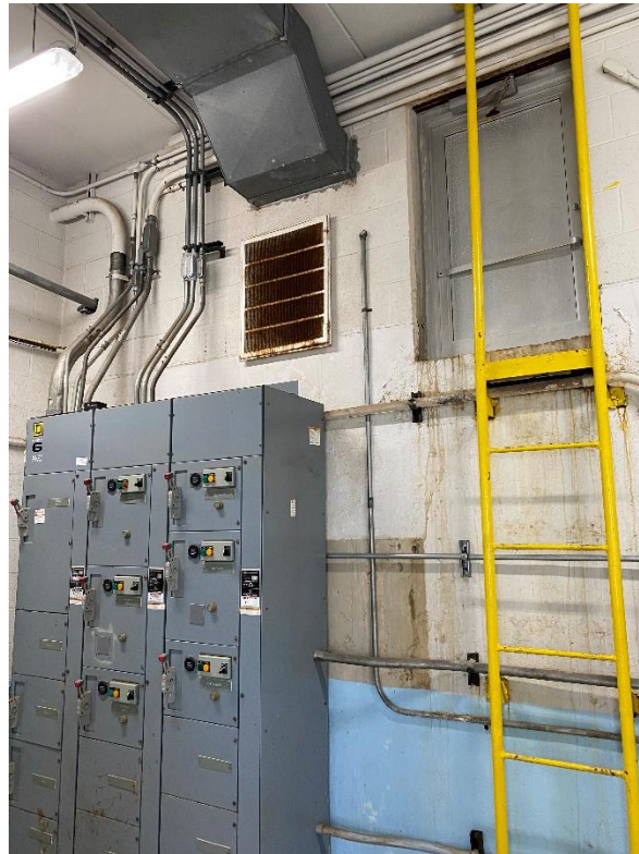
Figure 4: Access to Detention Tank
