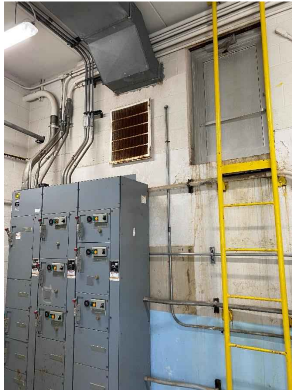
Figure 4: Access to Detention Tank
