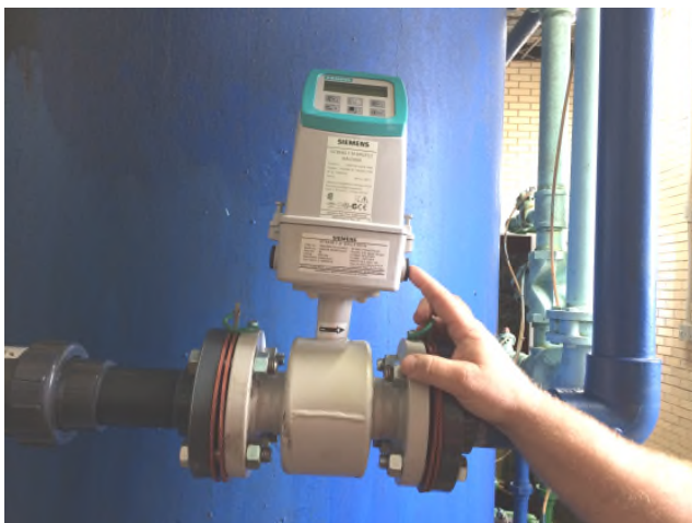
Meter 3 & 4 Inside With Control Attached
