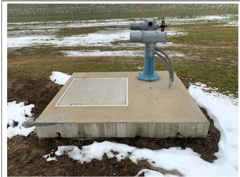
Figure 2.07.1 WAS Valve Vault Actuator Relocation
