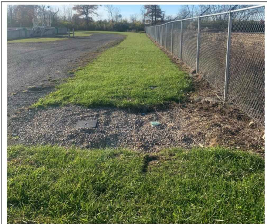
Figure 3.01-1 Existing North Stormwater Ditch
