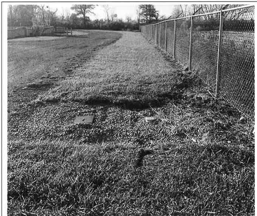
Figure 3.01-1 Existing North Stormwater Ditch
