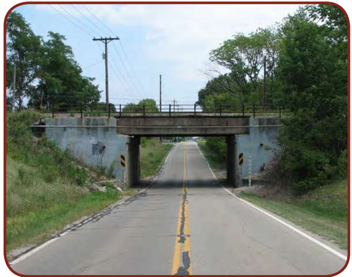
Fig 6-39 - Existing Railroad Overpass into Ashville (G2)
