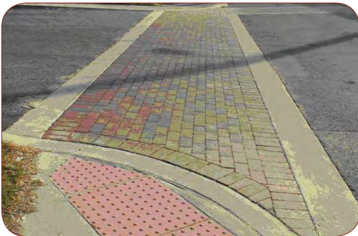
Fig. 7-9: A brick crosswalk. (Source: Higgins, Brian)
