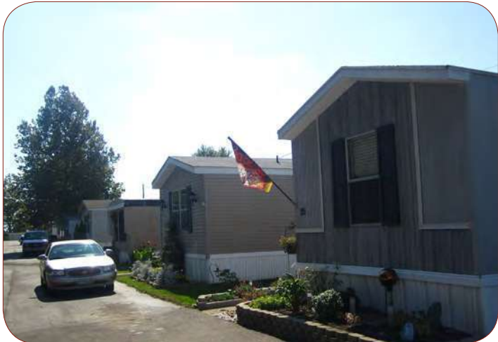
Fig. 2-15: Surveyed General Commercial Property - Mobile Home Park (Source: Urban Decision Group)
