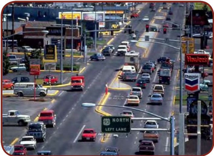
Fig 6-27 - Lack of Access Control or Pedestrian Accommodation
