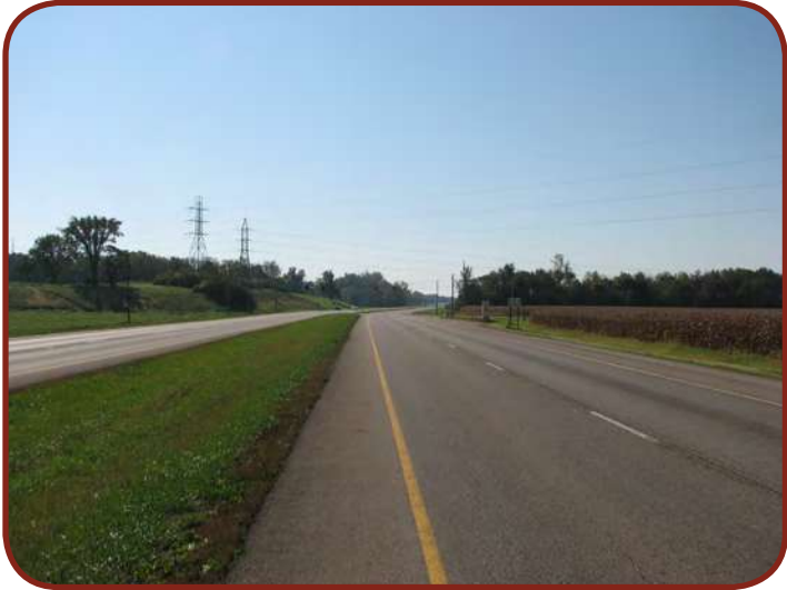
Fig 6-33 - Existing Character of US 23 (G2)
