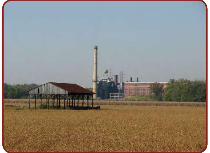
Fig 1-3 - Ex. Power Plant
