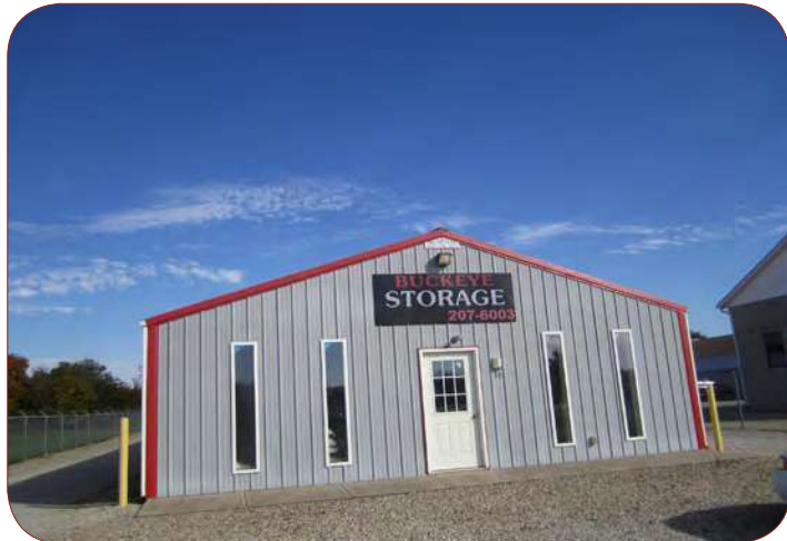
Fig. 2-17: Surveyed General Commercial - Storage Facility (Source: Urban Decision Group)
